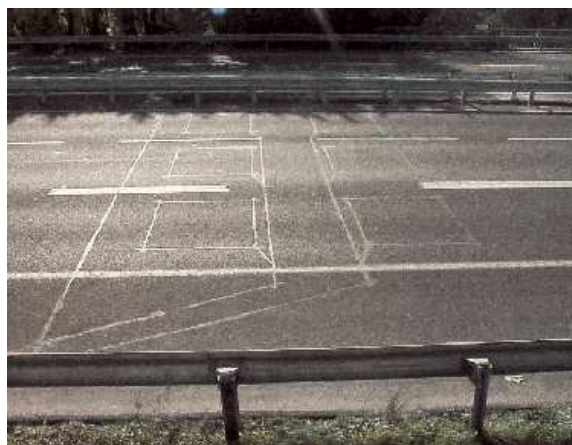
FIGURE 3.1 – Boucles inductives.
