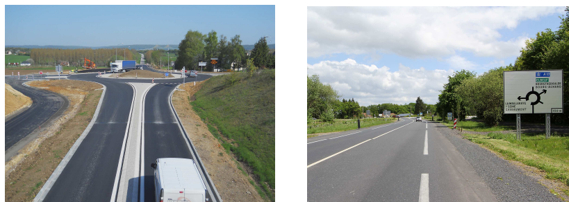
Fig. 3. (a) RD131-RD490 roundabout; (b) Passively safe sign posts (CG 76, 2013)
